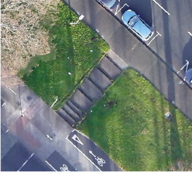
Figure 3.6: No tactile paving to indicate stairs
