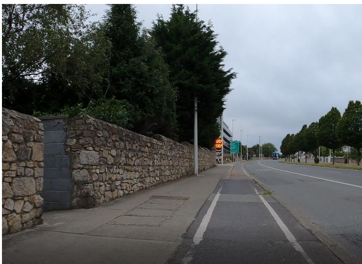
Figure 3.5: No level difference between footpath and cycle lane
