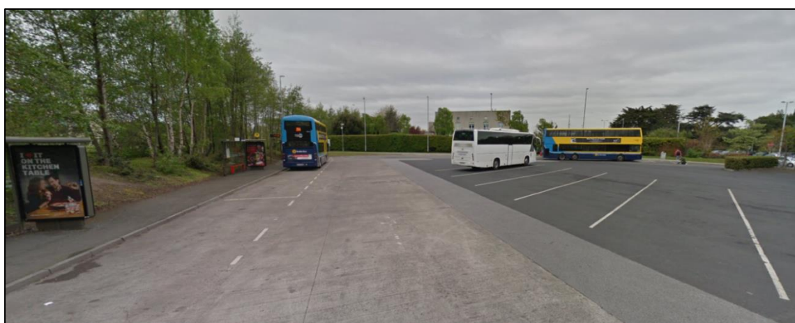
Figure 3.2: Photo of the existing bus terminus facility in UCD
