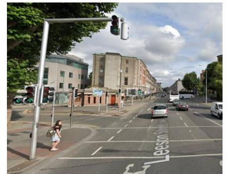
Figure 4.2 Cantilevered Signal Head on Leeson St Lower
