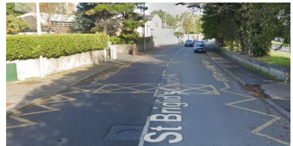
Figure 3.15 Road Markings outside St Brigid’s National School
