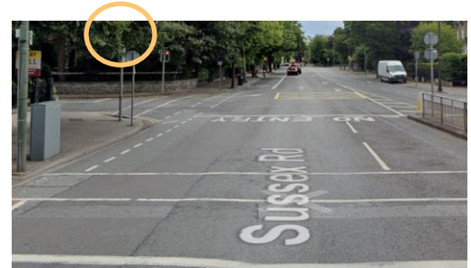
Figure 4.3 Visibility of signal head due to vegetation
