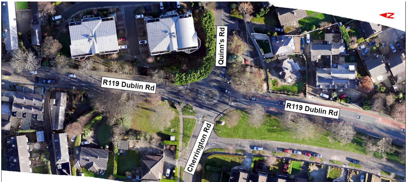
Image 6.40: R119 Dublin Road / Quinn's Road / Cherrington Road Four-Arm Roundabout
