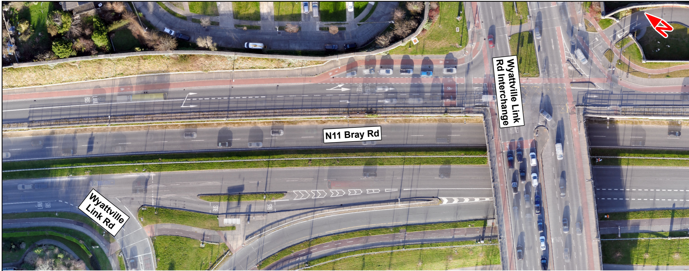
A) N11 BRAY ROAD NORTHBOUND / WYATTVILLE LINK ROAD INTERCHANGE
