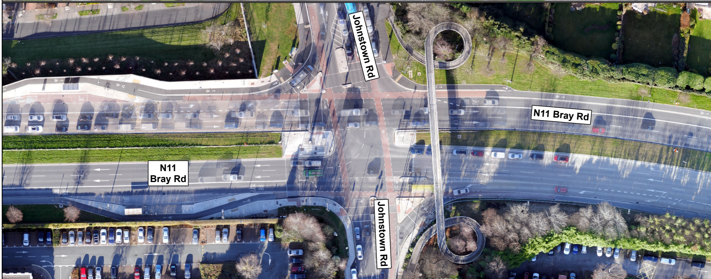
B) N11 BRAY ROAD / JOHNSTOWN ROAD
