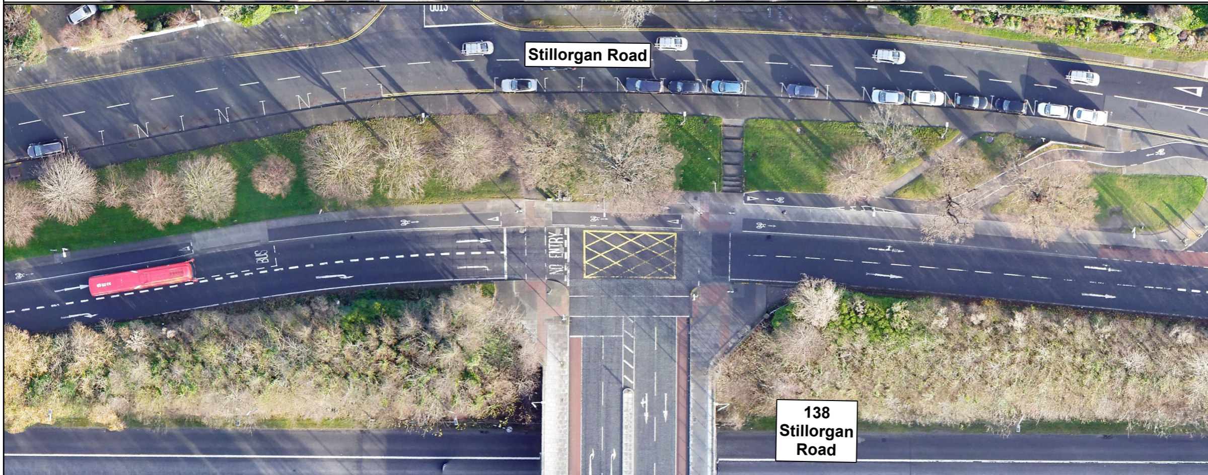
B) BELFIELD INTERCHANGE, SOUTHBOUND SIDE THREE-ARM SIGNALISED JUNCTION
