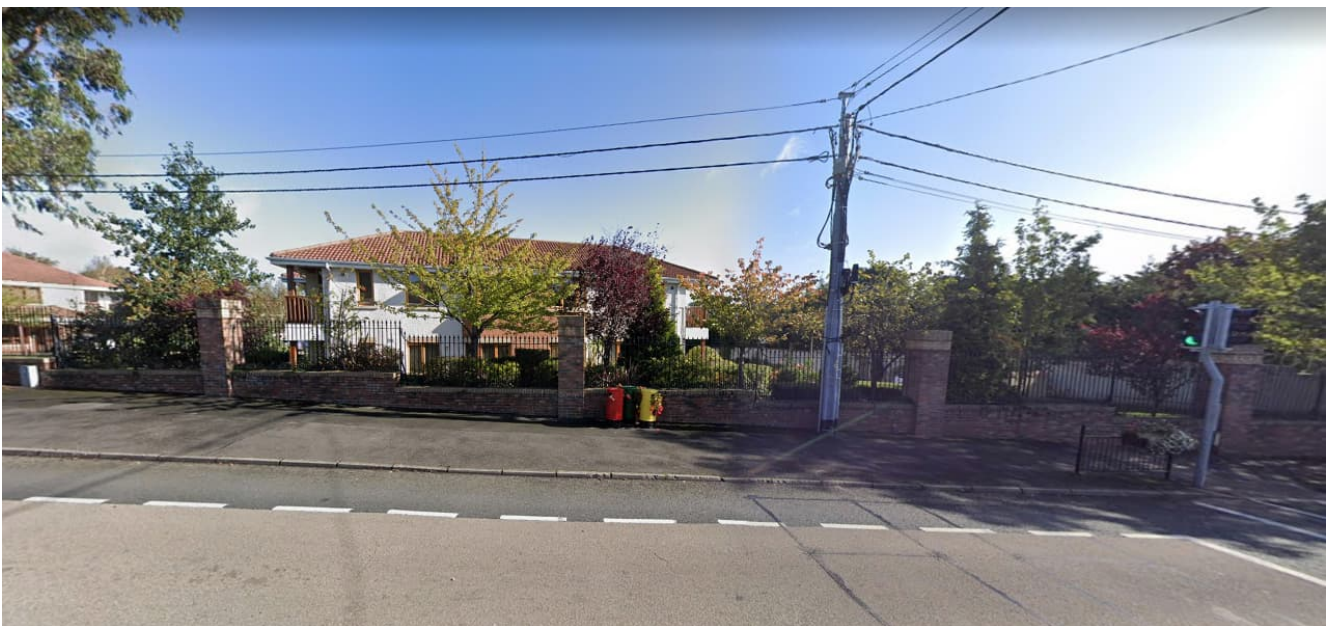
Figure 2.4.2: Photo of wall location R13-RW024
