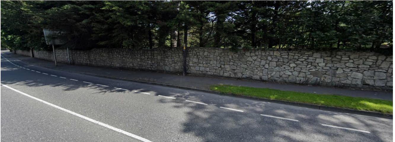
Figure 2.4.5: Photo of wall location R13-RW013
