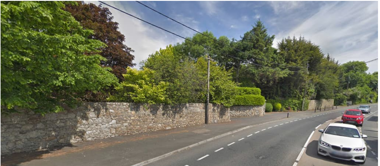
Figure 2.4.3: Photo of wall location R13-RW036
