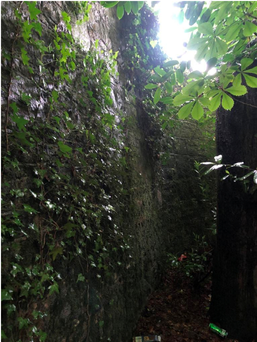
Figure 2 View of east elevation. Limited access
