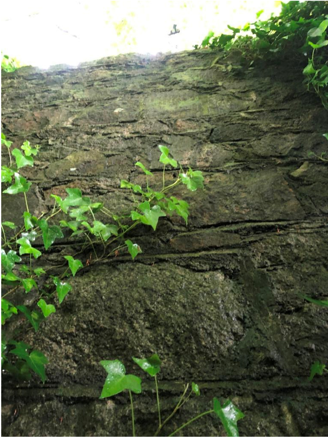
Figure 4 Typical condition of masonry on east elevation
