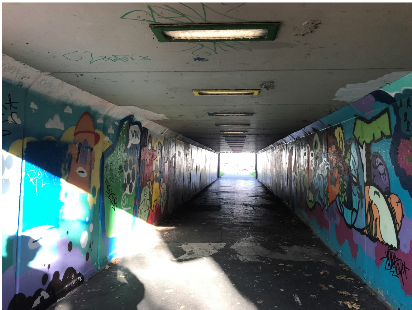
Figure 3.1: Interior of St Laurence Subway (November 2019)
