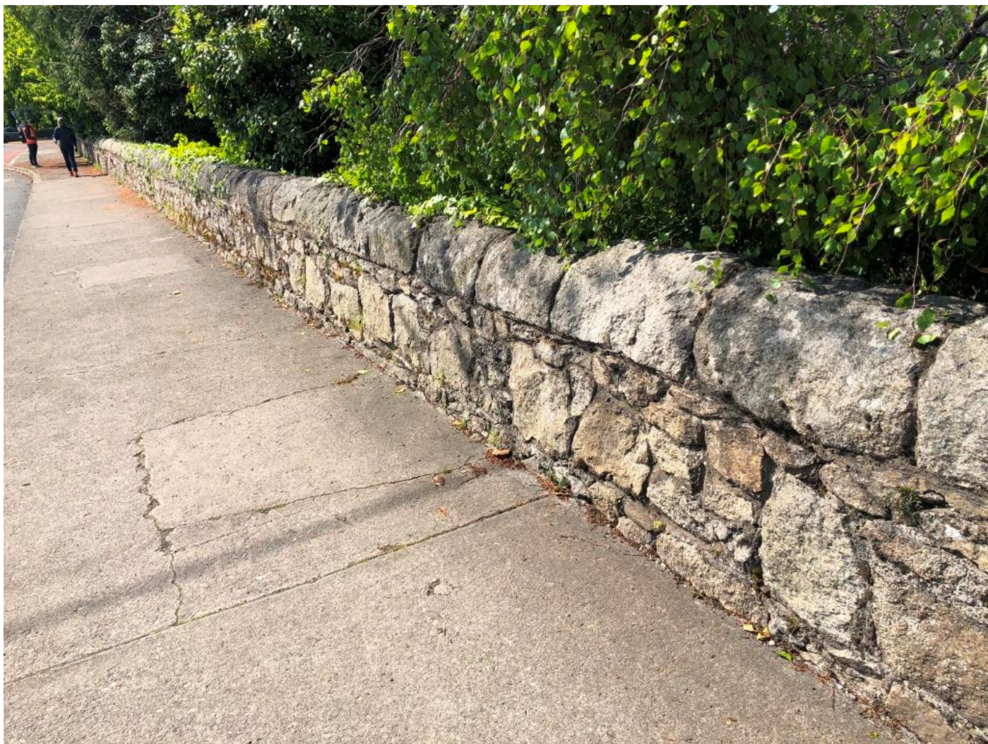
Figure 16 North west parapet in generally good condition.
