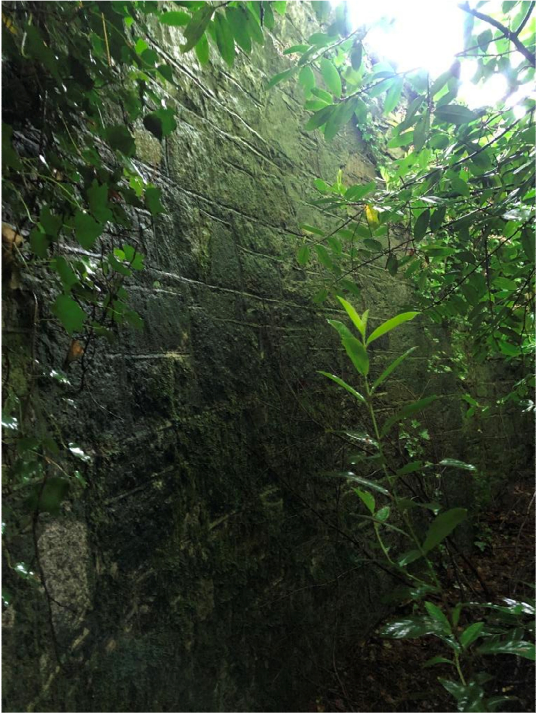
Figure 3 View of east elevation. Limited access
