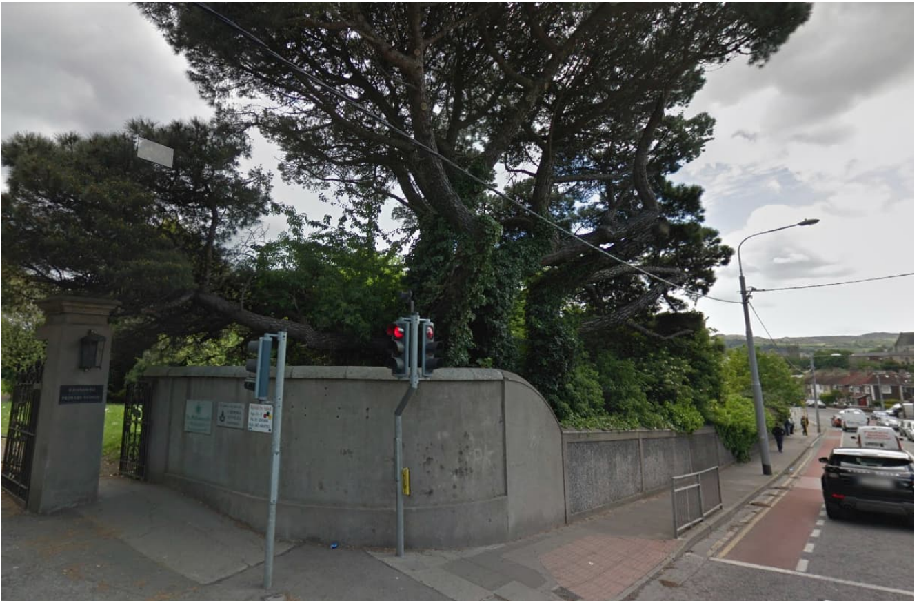
Figure 3.1.7a: Image of north end of R13-RW017 and the Monterey Pine Tree to be retained
