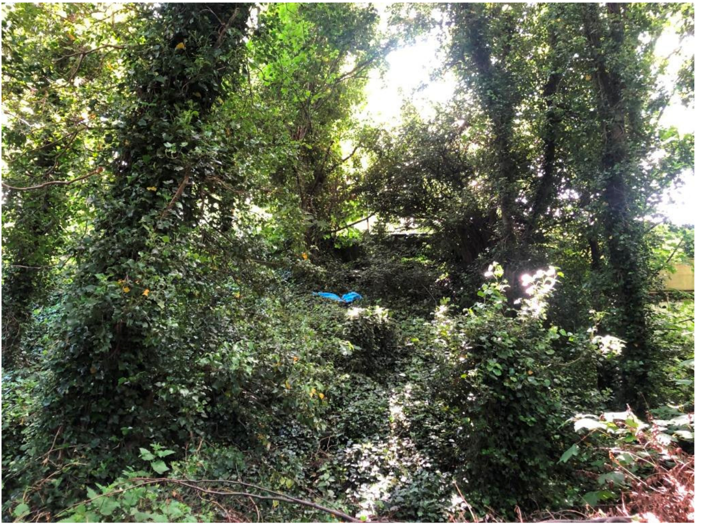
Figure 15 Extensive vegetation growth obscuring parts of the west elevation
