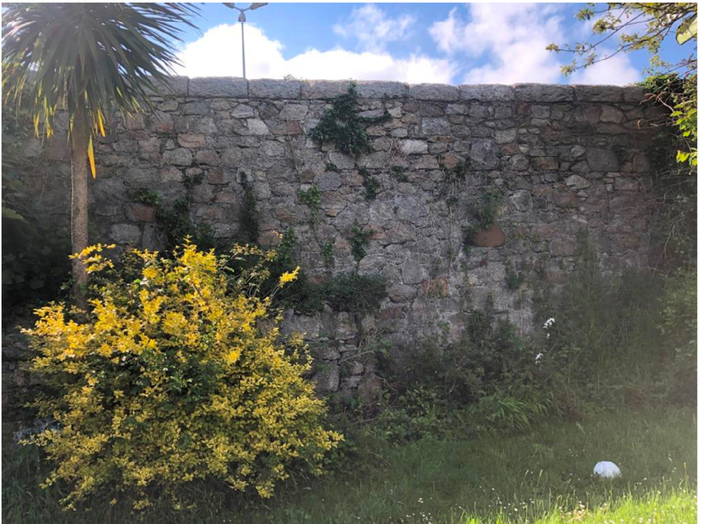
Figure 14 View of west elevation
