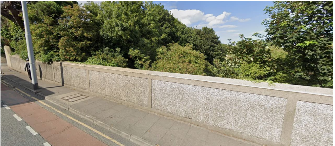
Figure 2.4.10: Photo of wall location R13-RW017
