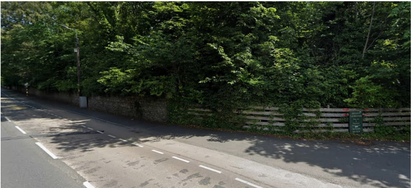
Figure 2.4.4: Photo of wall location R13-RW038
