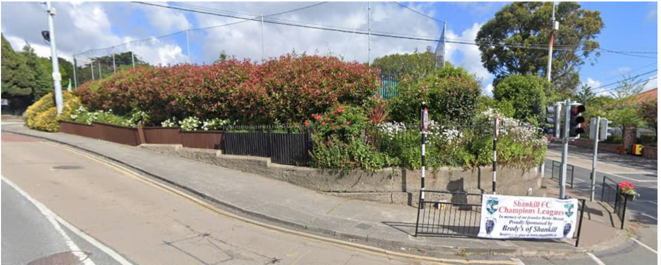
Figure 2.4.1: Photo of wall location R13-RW023
