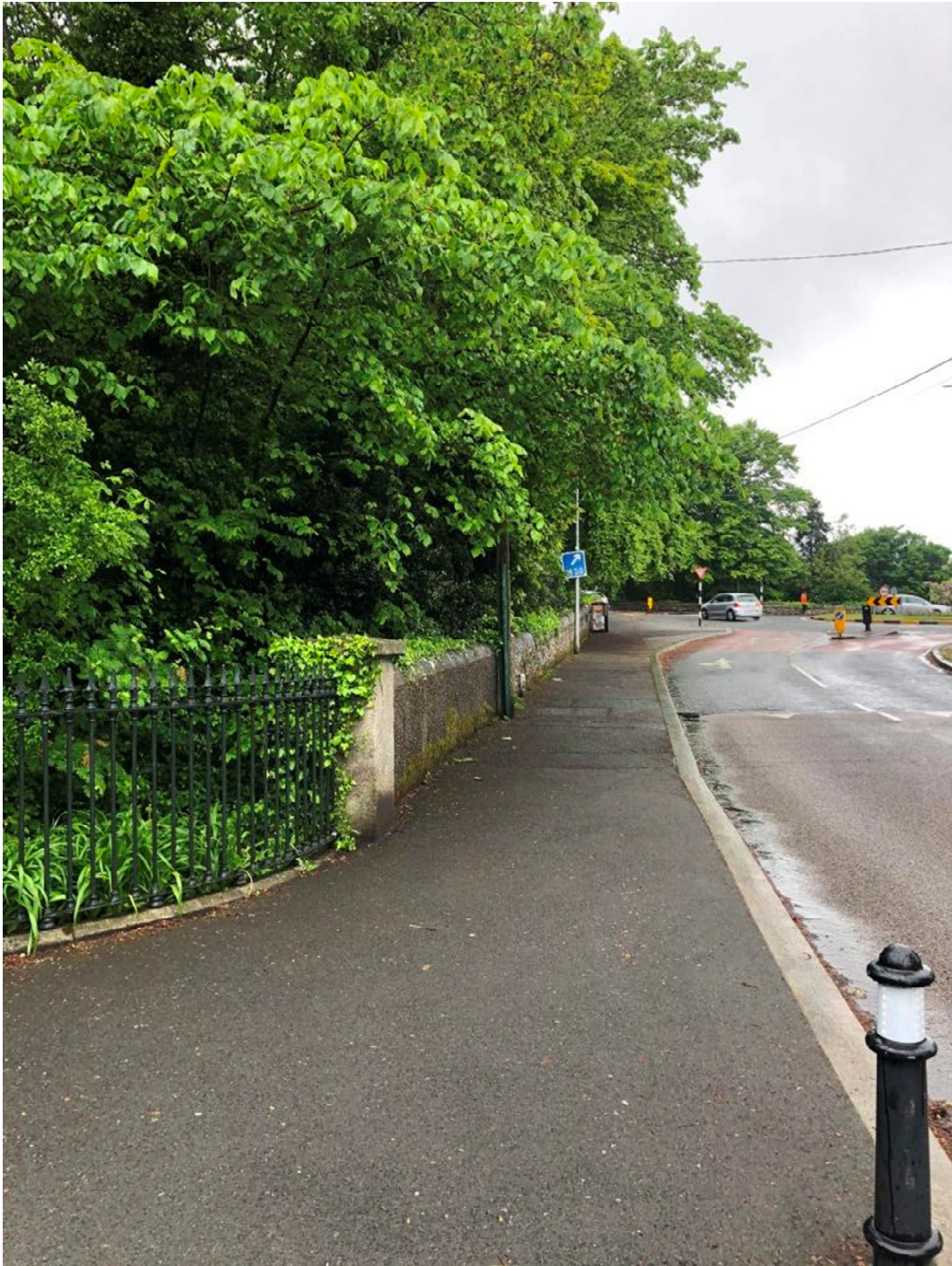
Figure 1 View of east wall looking north
