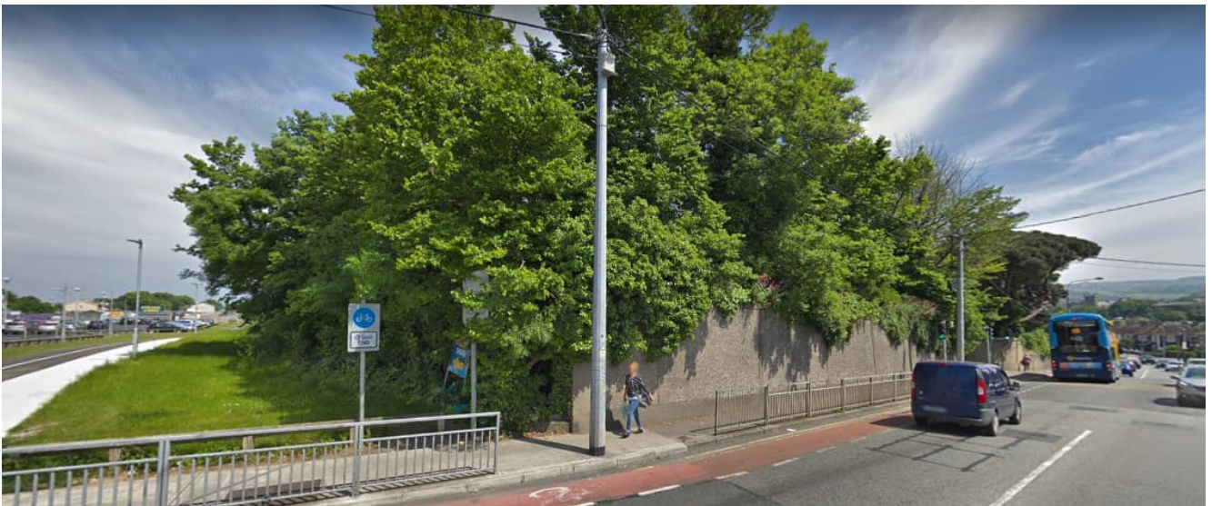
Figure 2.4.9: Photo of wall location R13-RW016
